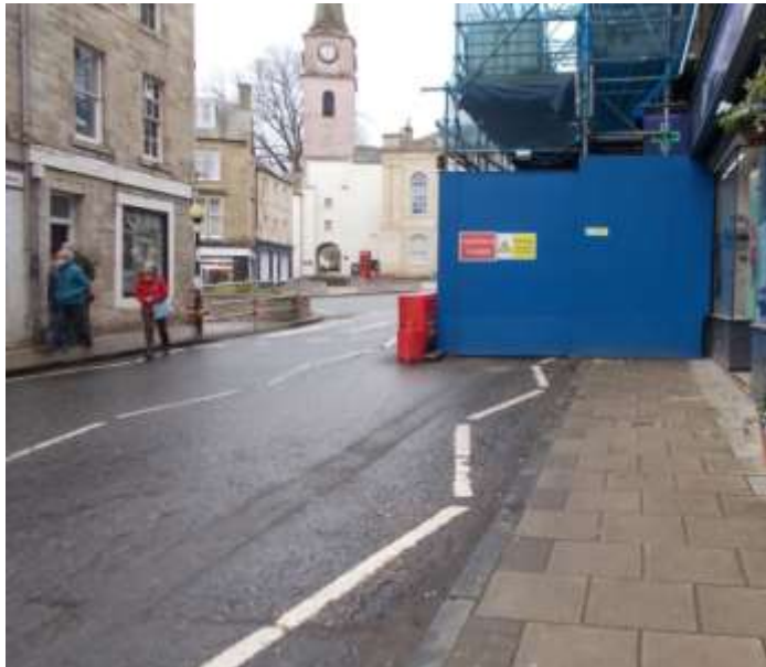
Termination of footway on High Street.
